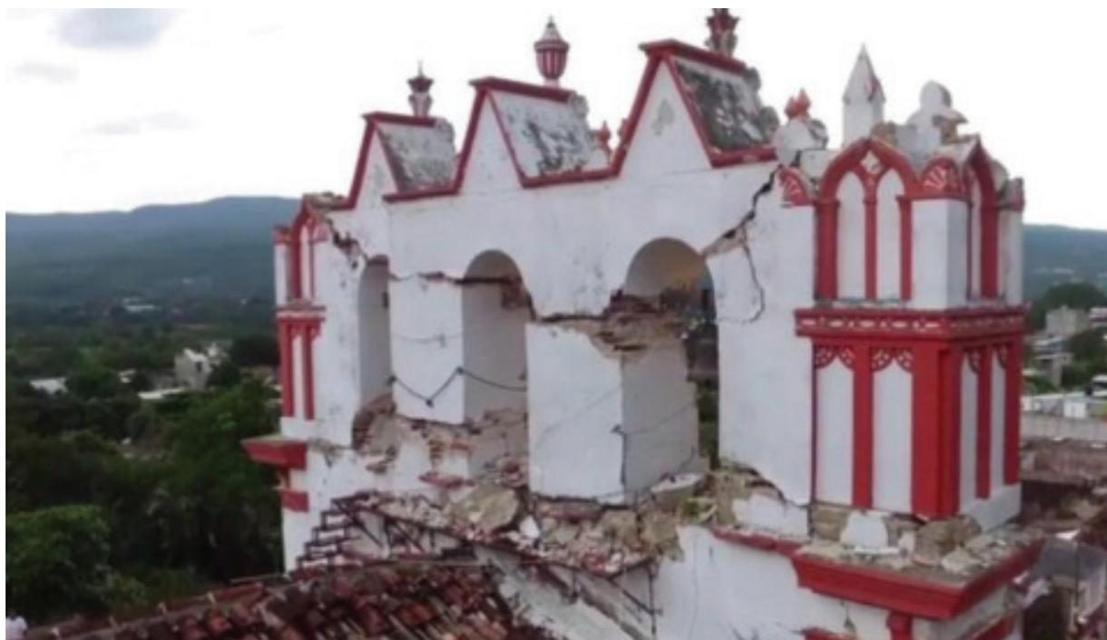
The damage to the roof structure of Capilla Sr. Del Calvario in Chiapa de Corzo in Chiapas. Photo courtesy of Fr. Carmelo Jimenez Salinas.
